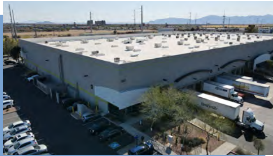
Chandler, AZ - Distribution Center
