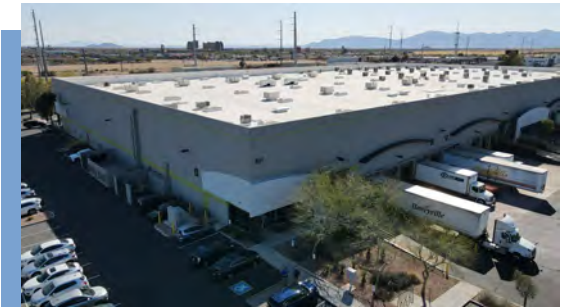
Chandler, AZ - Distribution Center
